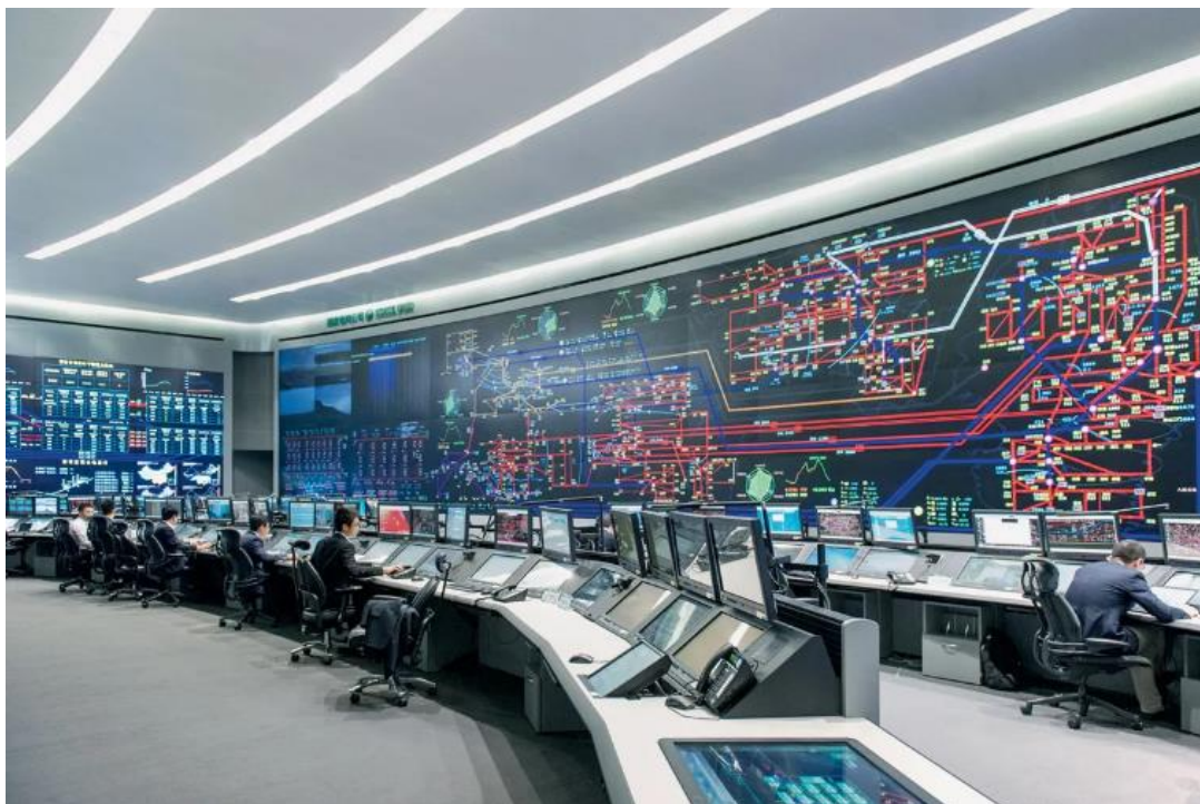
A dispatch centre in Beijing that controls most of China's ultra-high-voltage lines and monitors renewable electricity inputs. Photo from State Grid Corp of China
